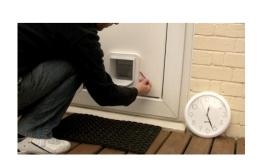
You will need to cut a larger hole in your door – leaving a gap of 2-3cm between the tunnel of the SureFlap and the metal in your door. To start with trace around the back frame as a good guide size.
