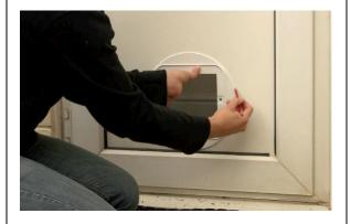
Using the SureFlap mounting adaptor as a guide trace around the circumference of the circular mounting adaptor.
